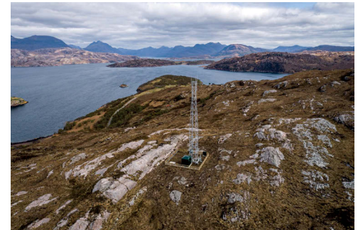
Masts in place at (top) Polbain and Kenmore (bottom)
